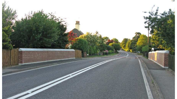
The New Chipping Bridge
